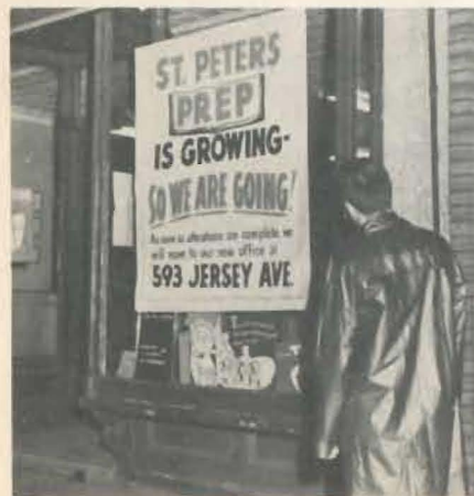
Prep is tearing down the store.
